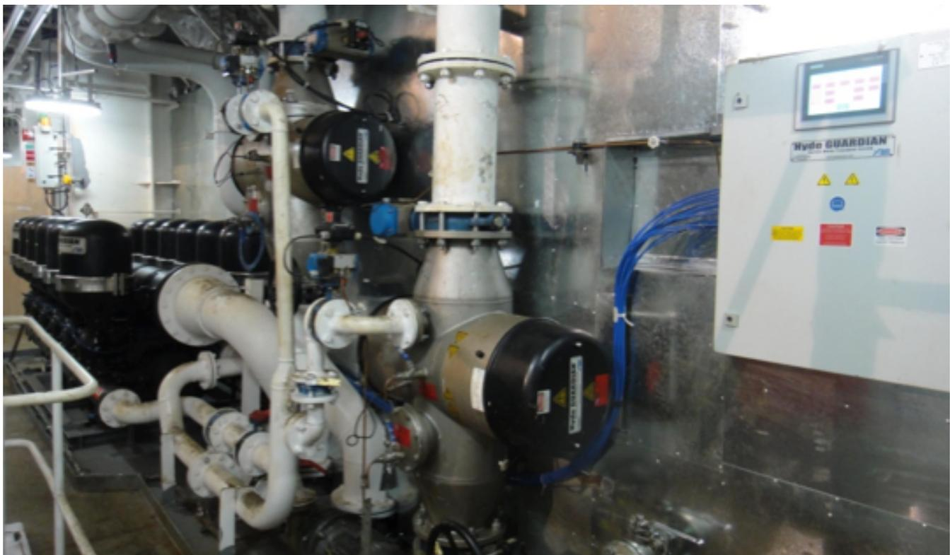
Hyde GUARDIAN installed aboard a bulk cargo vessel. Shown is the filtration system, two UV chambers, and the controller. System capacity: 500 m<sup>3</sup>/hr.
