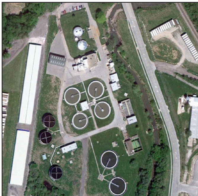
Figure 1: City of Leavenworth, KS wastewater treatment plant.
