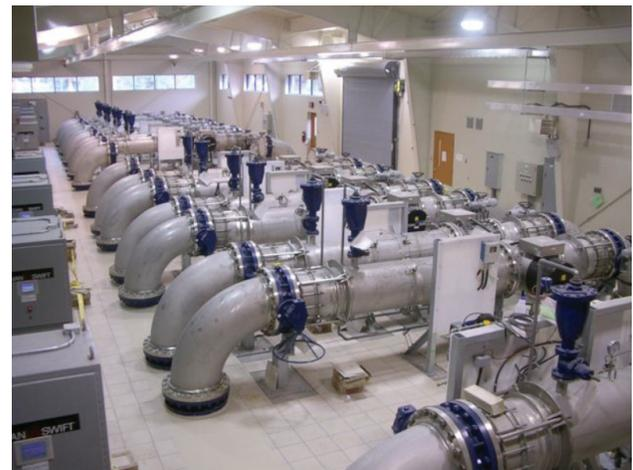
Figure 4. UV reactors and headers installed
