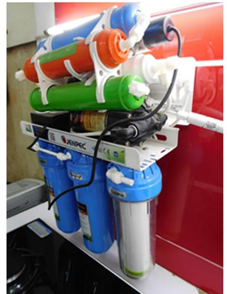
**Figure 2.** A multicartridge POU apparatus commonly found at households in Hanoi
